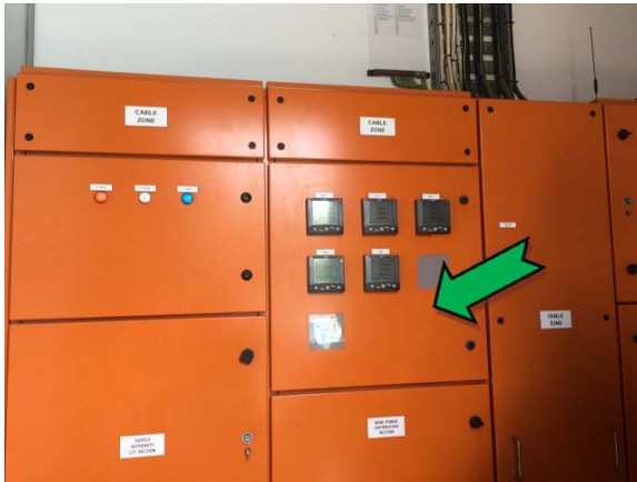
Photo 3. Interior, main switchboard room – suspected non asbestos-containing bituminous backing board.
