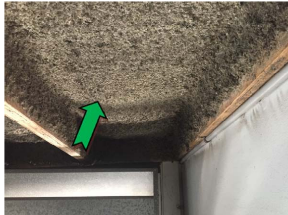
Photo 2. Interior, air conditioning plant room, ceiling – non asbestos-containing vermiculite.
